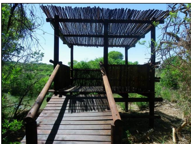
The bird-hide with its new roof, that offers some protection from the sun and will make people on the deck less visible.
