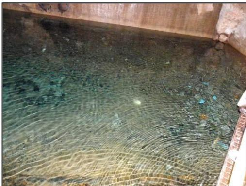
Thin streams of water can be seen coming through the sand under the water. The water from both fountains goes to a Mixing Chamber and then to supply the city centre.
