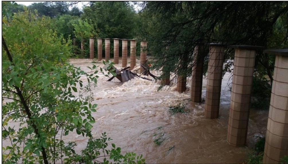
Water flowing past the flood attenuation structure upstream of the January Masilela bridge in Faerie Glen Nature Reserve on 23 March. The high water mark can be seen on pillars. (Photo: Edwin van de Wiel)
